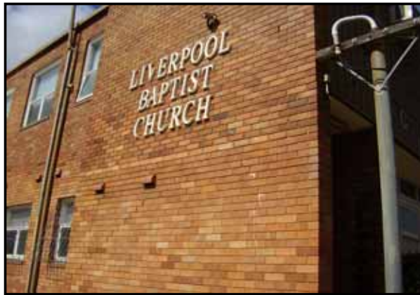
Photo 2 Two storey brick church building
