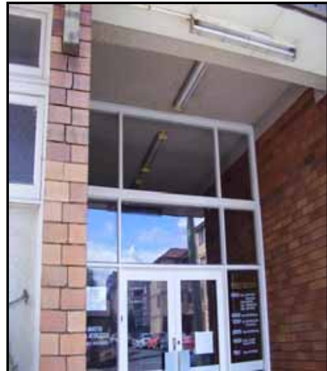
Photo 3 Entrance to two storey church building
